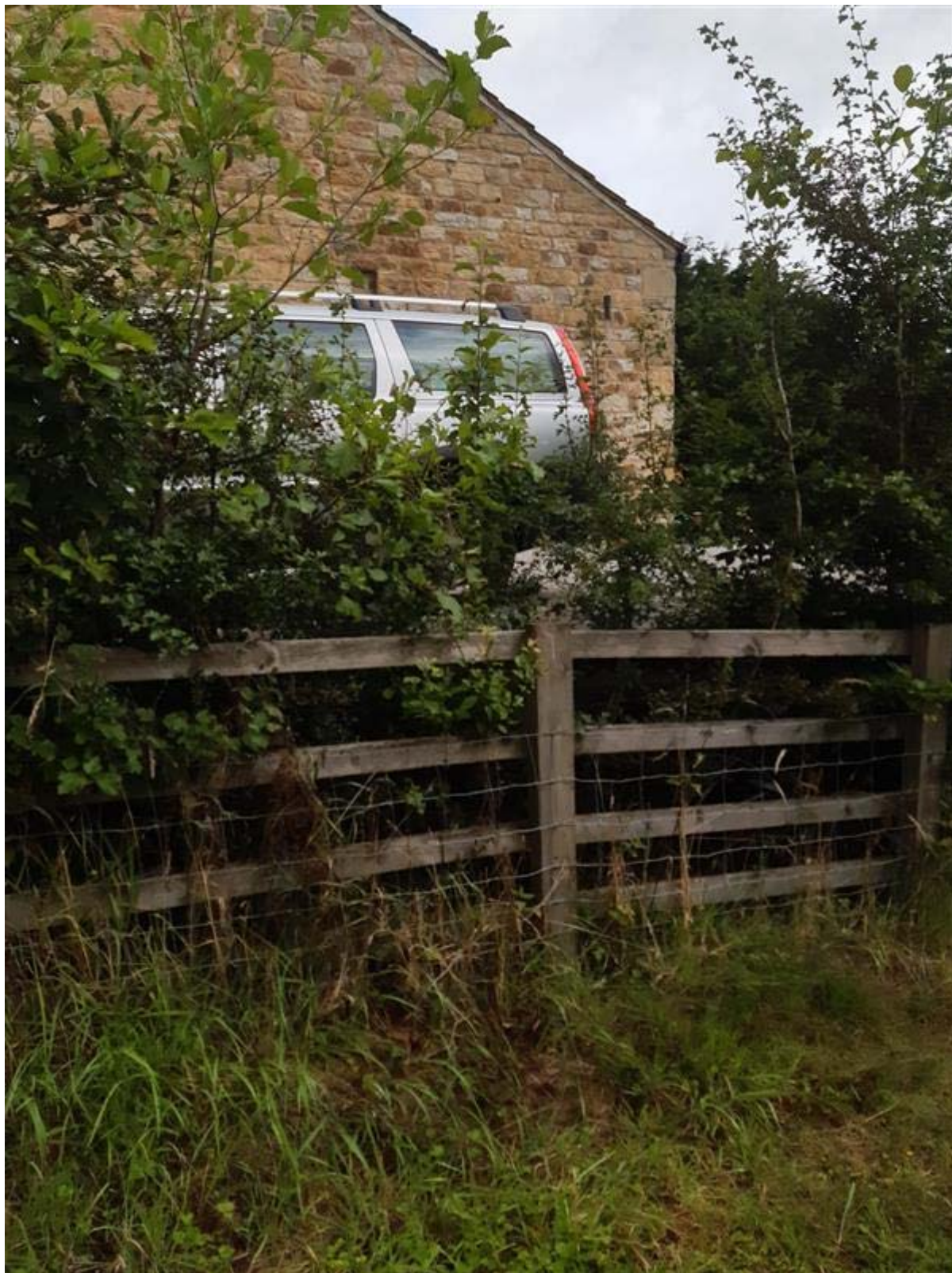
Photo 2 - Fullwith Mill Farm Gable
