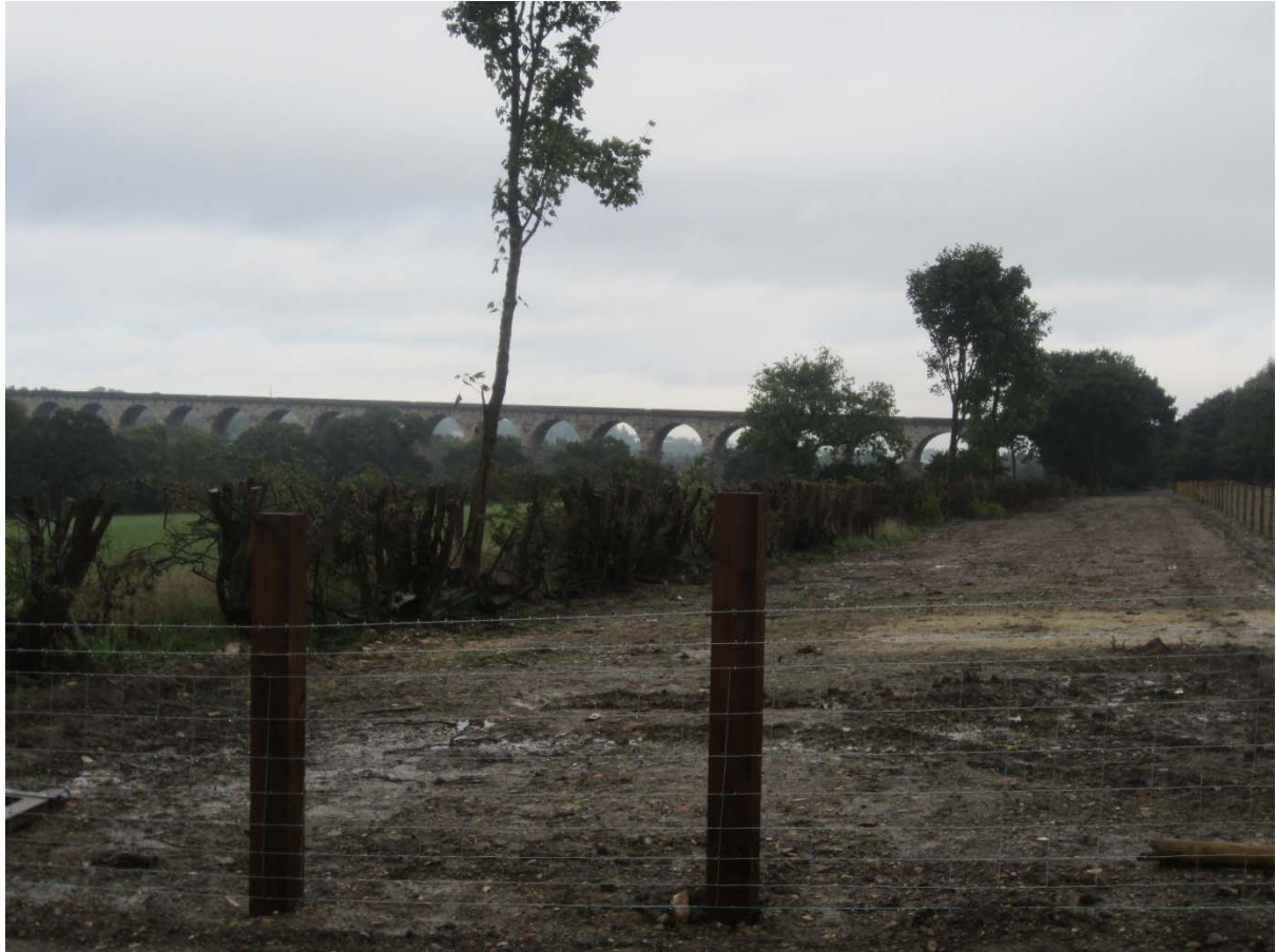
Photo 8 – Looking east along new bridleway on old railway line
